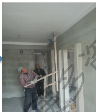
膨胀螺栓开孔
