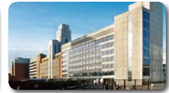
MITIE Infrastructure Ltd(英国)
